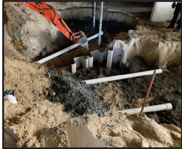
Figure 4: Soil Mixing and Injection Laterals
